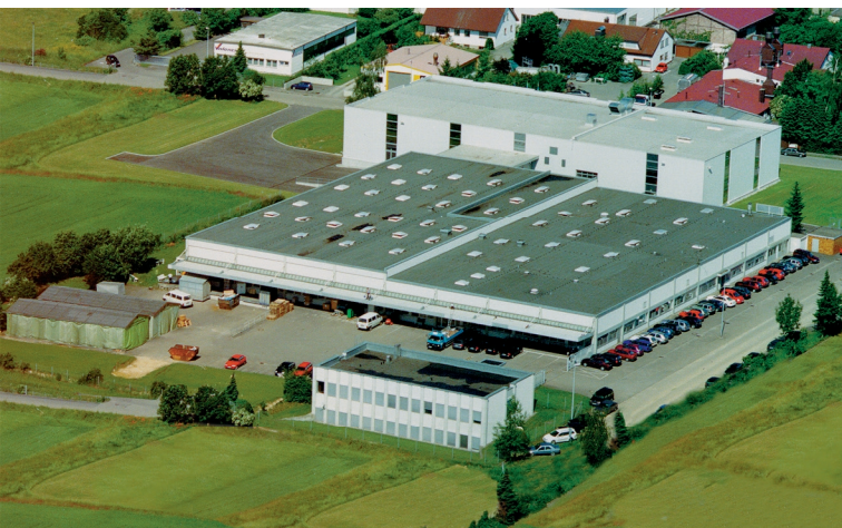
offices and factory in Langenau
